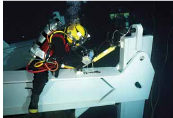
Figure 30. A saturation diver working on the turret support structure during the turret recovery from the USS Monitor. Photo by Eric Lippmann.
